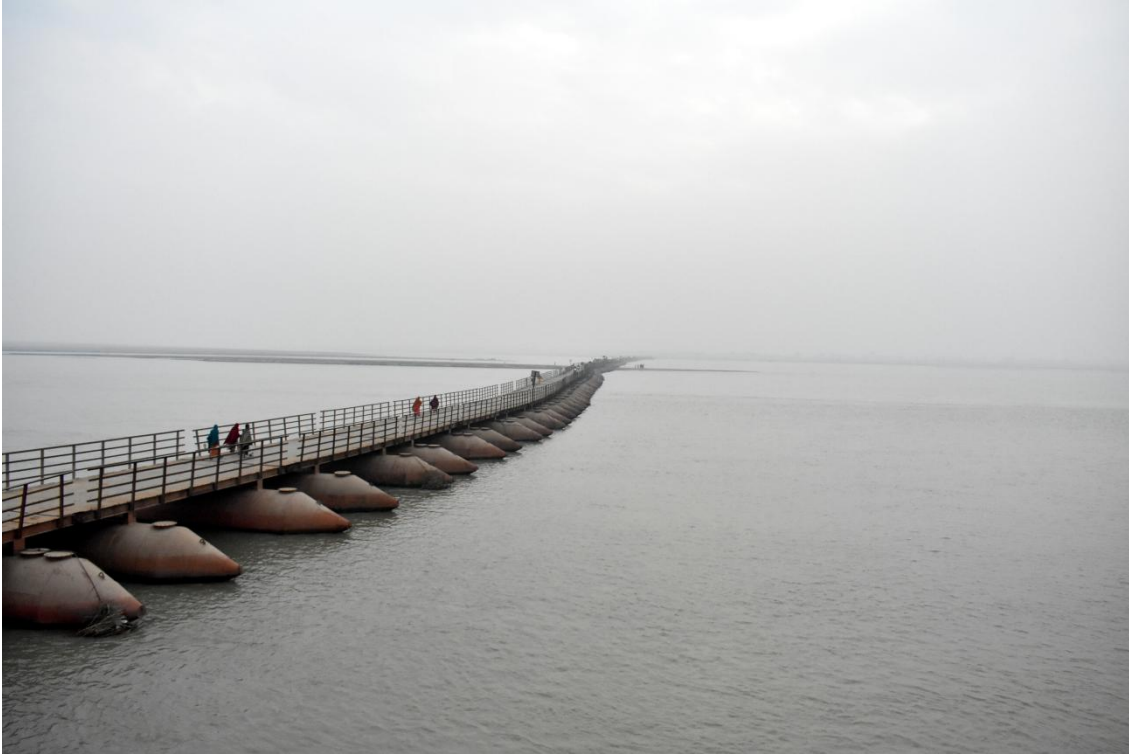
Image 30 : A Pontoon Bridge Connecting Raghapur Diara With Vaishali Distt.
