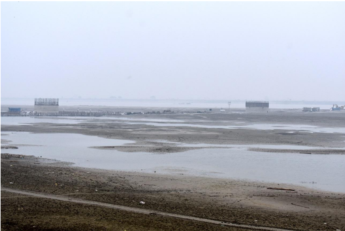
Image 31 : A New Bridge Being Constructed To Connect Raghapur Diara With Vaishali Distt.
